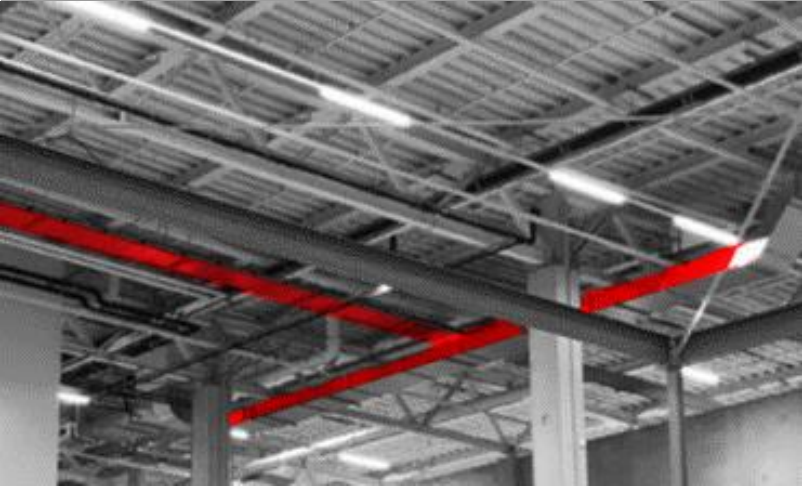
Power and data cable pathway management
