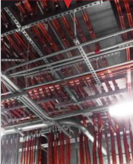
Fire rated wiring and leak detection
